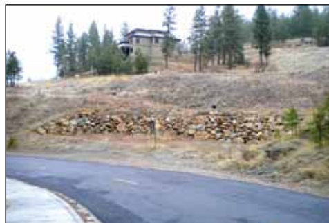
Retaining wall constructed of Hauser Lake Gneiss
